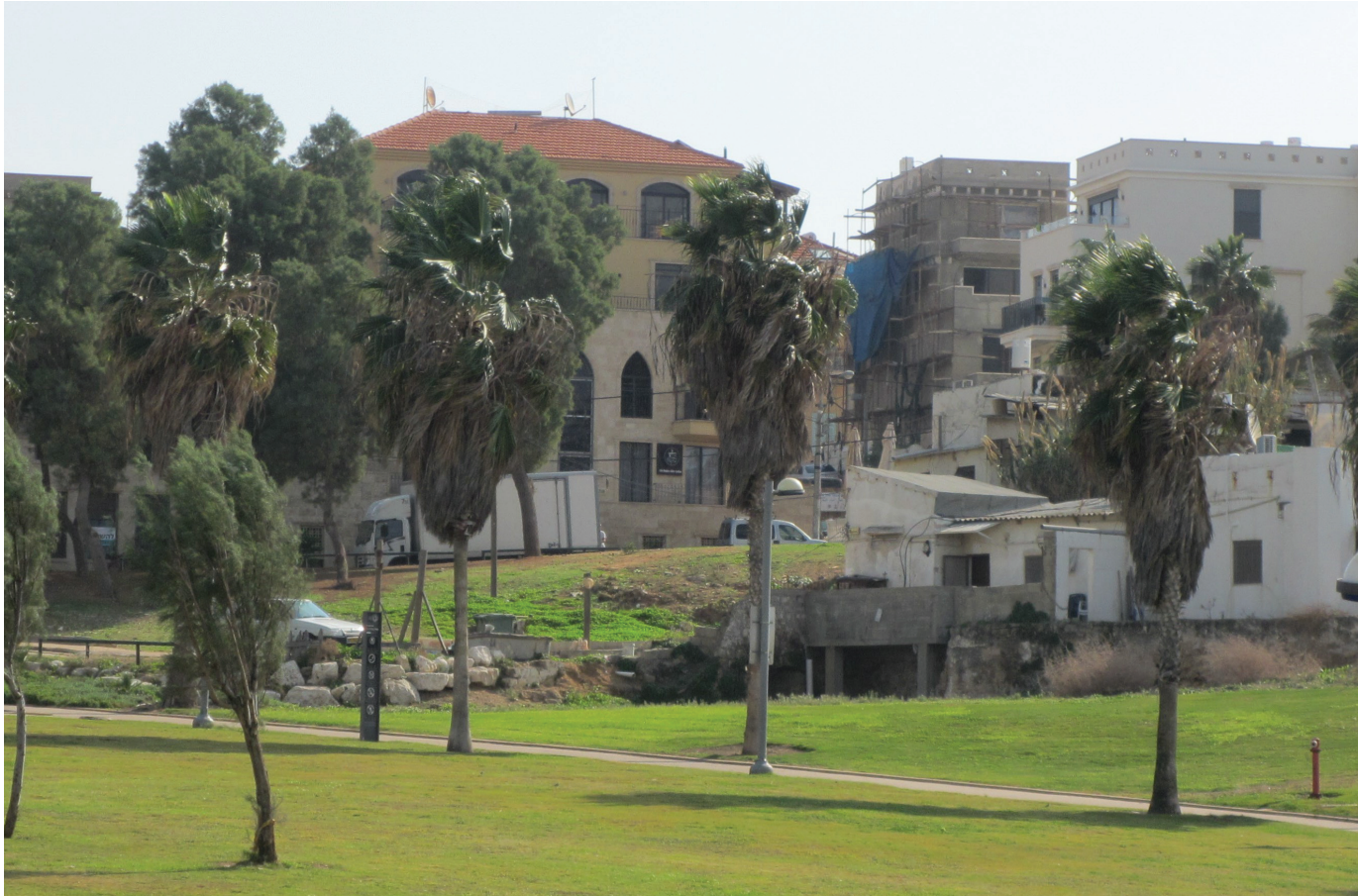
FIGURE 6 Landscape of green gentrification. Ajami neighbourhood homes at the eastern thresholds of Jaffa Slope Park: Old Palestinian home in the front; renovated or new buildings at the back, which use all the building rights that the valid urban master plan added (Image by author, 2018).
