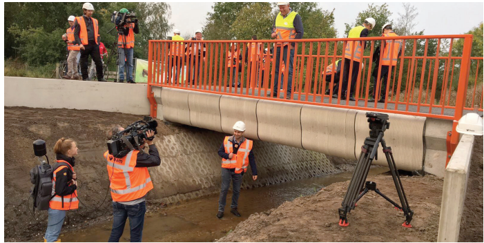
FIGURE 7 The world's first MDM-printed concrete bridge for bicycles in Gemert, Noord Brabant, on opening day. The printed layers contain steel cable as lateral reinforcement (the bridge is prestressed in the longitudinal direction).
