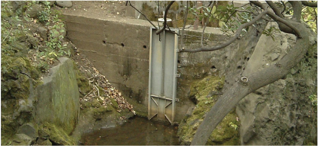
FIGURE 7 The inlet point of garden pond from the river, in old Yasuda garden, Ryogoku, Tokyo
