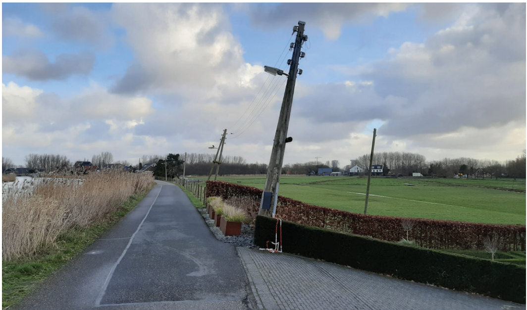
FIGURE 4 Telephone poles along the Rotte. In Chabot's monumental paintings, slightly slanted telephone and lantern poles appear again and again. They attach the land and the sky, and direct the eye to the distance. These poles appear here and there along the Rotte and indicate very precisely the amount of subsidence of the land. (Photo by Observatorium, 2020)
