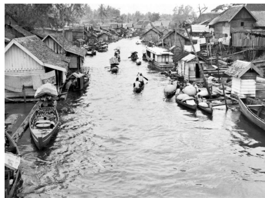
FIGURE 4 Riverscape in the past | Floating structures and lively activities on the water, 1920-1940. National Museum of World Cultures, Collection Tropenmuseum.
