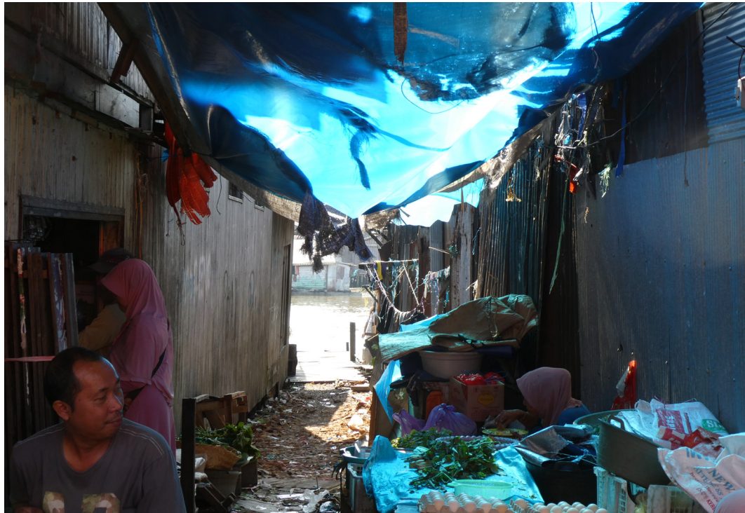
FIGURE 10 Changing focus of riverine settlements | Pasar Lama's alleys connecting the market streets with the river are barely used anymore.
