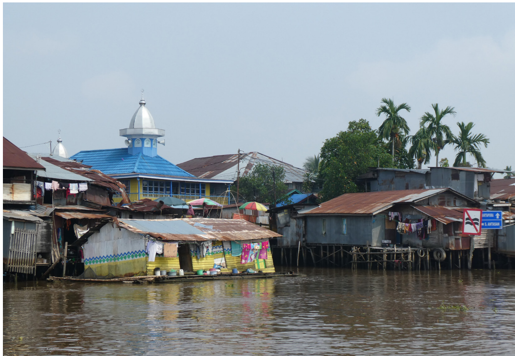
FIGURE 7 Building typology of riverine houses | Stilt houses and a floating house (left) at the junction between the Martapura and the Kuin rivers.
