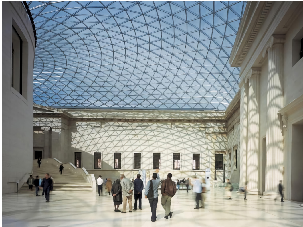
FIGURE 3 The Great Court Roof grid-shell of the British Museum form-found by Chris Williams (image credits: Foster + Partners, Nigel Young).
