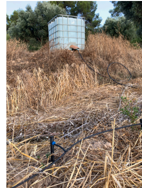
FIGURE 21 System of hoses
