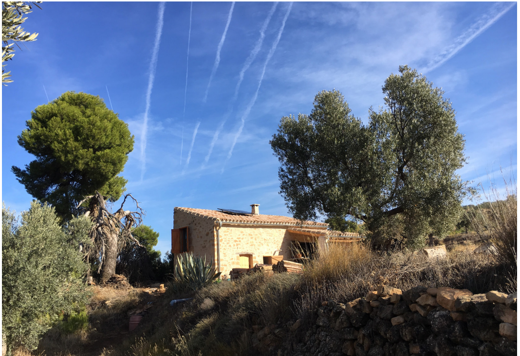
FIGURE 10 The barn after renovation
