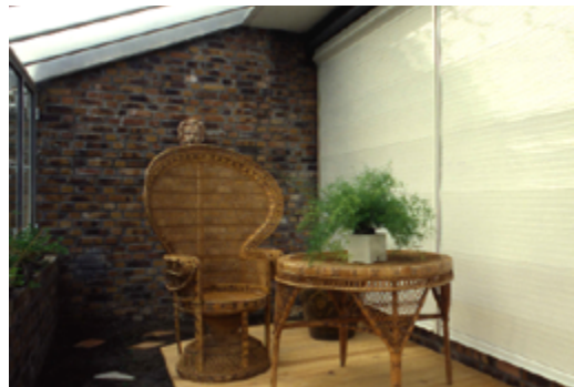
FIGURE 13 Maison particulière, Internal view of the greenhouse. Detail of the (white) rotating shutter closed in front of the thermal mass wall. (Image by Marc Vaye © , 1980)
