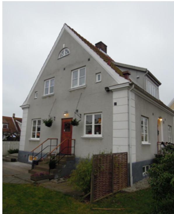
FIGURE 3 The neo-classical villa to which Unit C was added.
