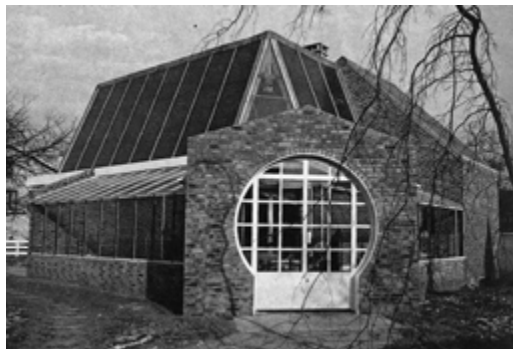
FIGURE 12 Maison particulière, Argenteuil, Val d'Oise. Main entrance on the south. (Techniques et architecture, 6/1979)
