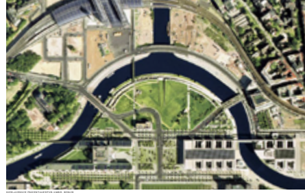
This aerial photograph offers a good overview of Spreebogenpark. In the north the brand new Hauptbahnhof is in the south the strip of government buildings that separate the Spreebogenpark from the Potsdamer Platz. The green space in front of the Reichstag.
