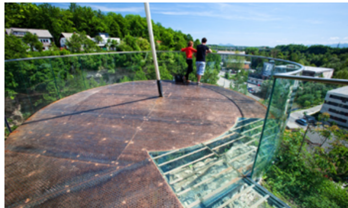
FIGURE 8 The view from the platform. The perforated surface and walk-on glass expose the medieval wall and the height of the slopes. This is one of the rare places where the river gorge and the height difference between the city and its surroundings can be observed. By also offering long vistas it is a key point for understanding the city's context. (photography by Luka Dakskobler, arhiv Zavoda za turizem in kulturo Kranj, 2016).
