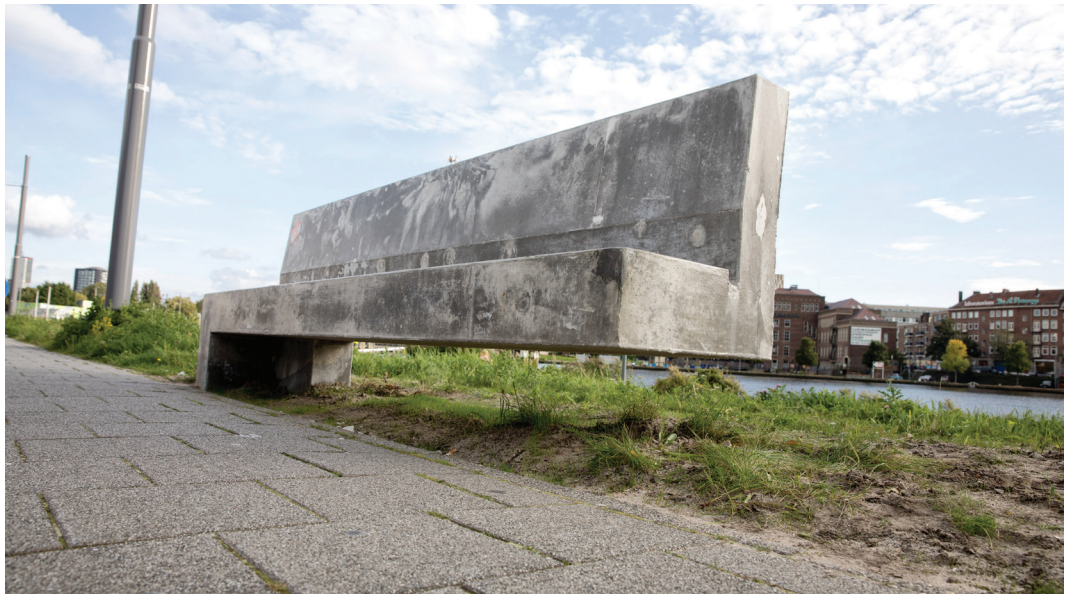
FIGURE 8 Reinforced geopolymer concrete bench made of the optimized geopolymer concrete mixture. The bench has been located in the street G.J. de Jonghweg, Rotterdam.
