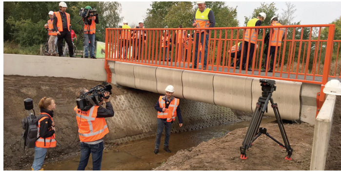
FIGURE 7 The world's first MDM-printed concrete bridge for bicycles in Gemert, Noord Brabant, on opening day. The printed layers contain steel cable as lateral reinforcement (the bridge is prestressed in the longitudinal direction).
