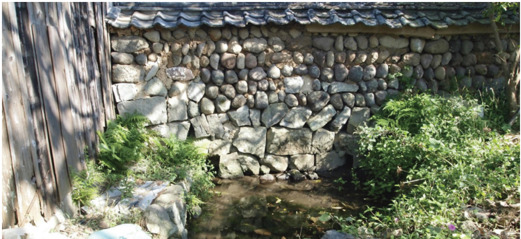
FIGURE 12 Garden pond with piled stones wall to prevent to flooding.
