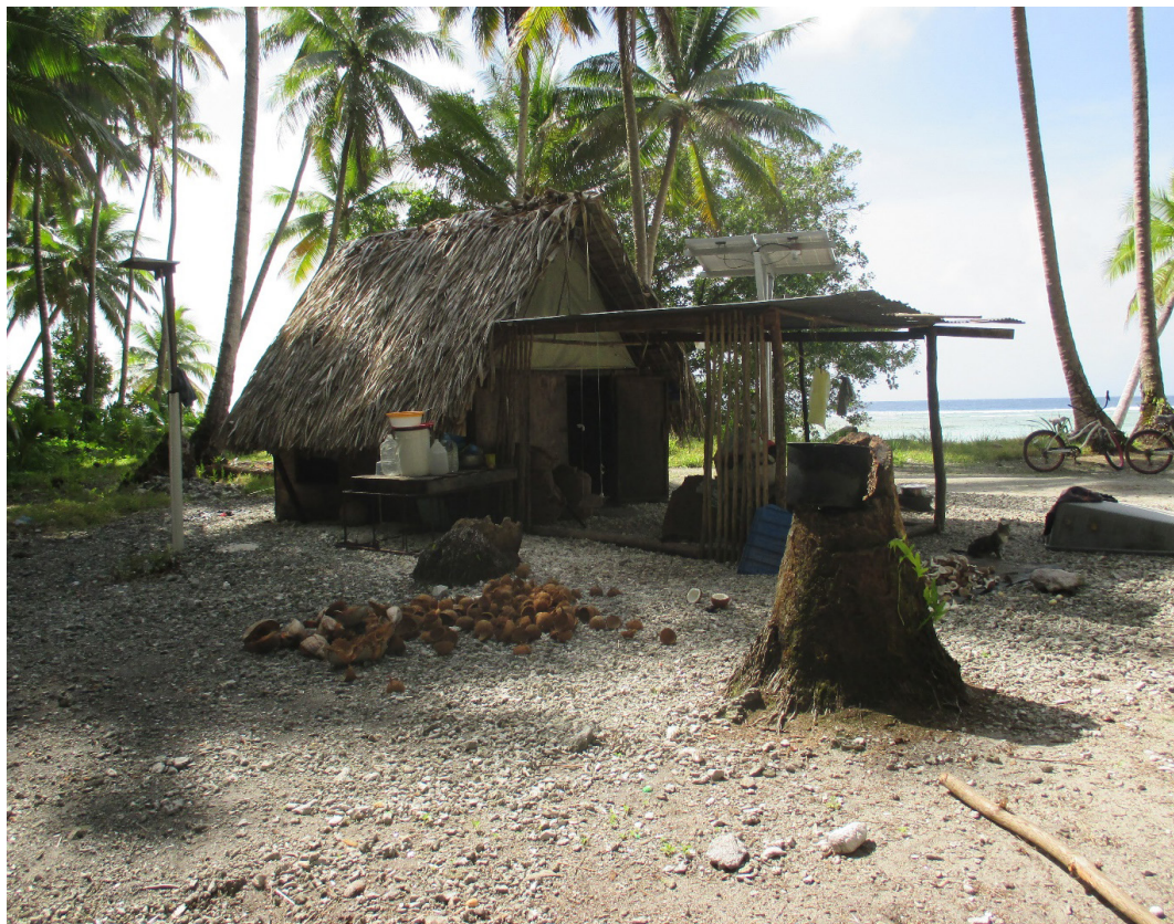
FIGURE 1 Photograph of a modified monkijdrick on Namdrik Atoll. This dwelling demonstrates similar material use and structural design to the monkijdrick, but has closed exterior walls as opposed to four posts. Photo by author.
