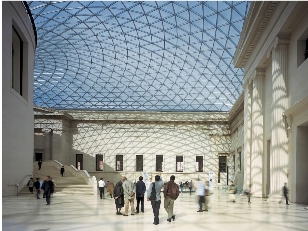
FIGURE 3 The Great Court Roof grid-shell of the British Museum form-found by Chris Williams (image credits: Foster + Partners, Nigel Young).
