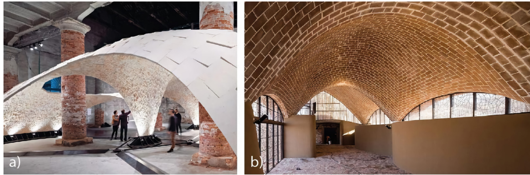
FIGURE 4 a) The mortar-less 'armadillo' vault as exhibited at the Venice Biennale in 2016 (Block et al., 2017); b) The long-span shell of the Mapungubwe National Park comprising structural tiles (image credits: Iwan Baan).
