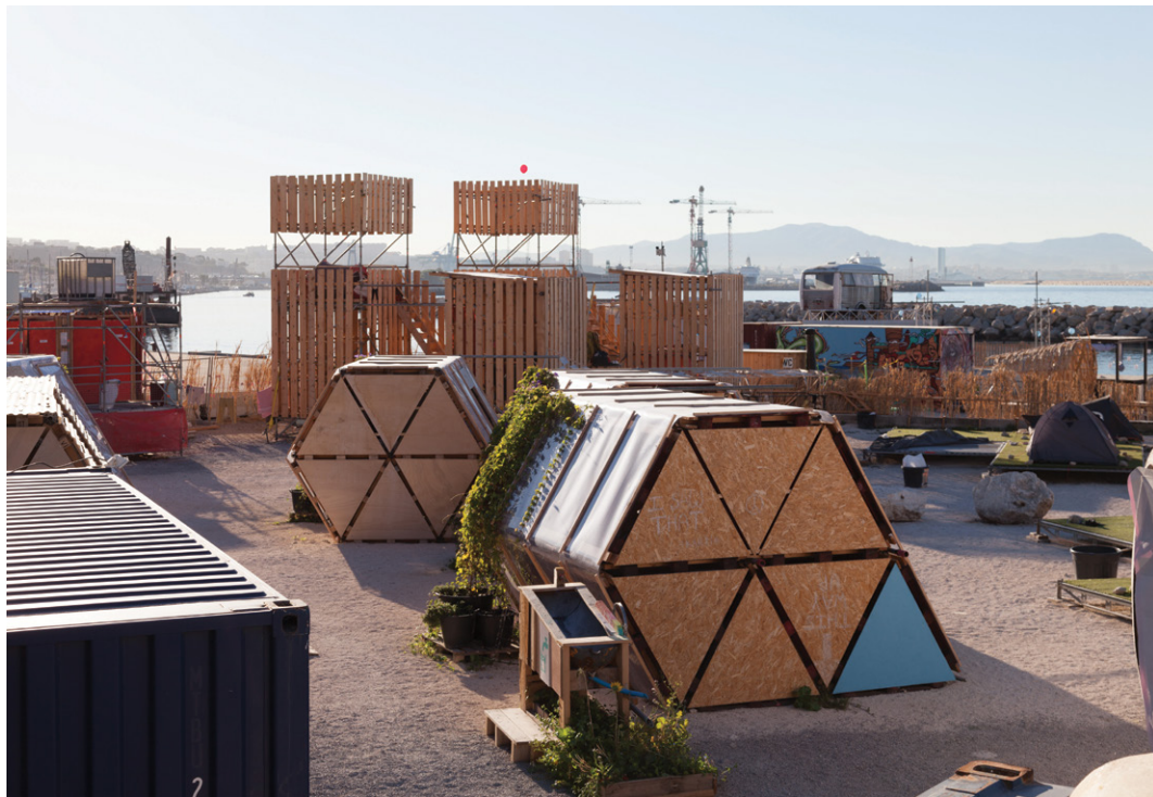
FIGURE 4 'Moissonneuses' - 'Combines' on the front and Perched Huts in the background. Dorms and small rooms built on scaffolds made out of wooden materials and recycled pallets and 'Les Cabanons perchés' (Perched huts) two-storey perched and shady platforms for tents built on scaffolds are among the flagship constructions of the camping. Designed by BC Architect & Studios and Michael Lefeber. (Photograph by Yes We Camp! 2013).
