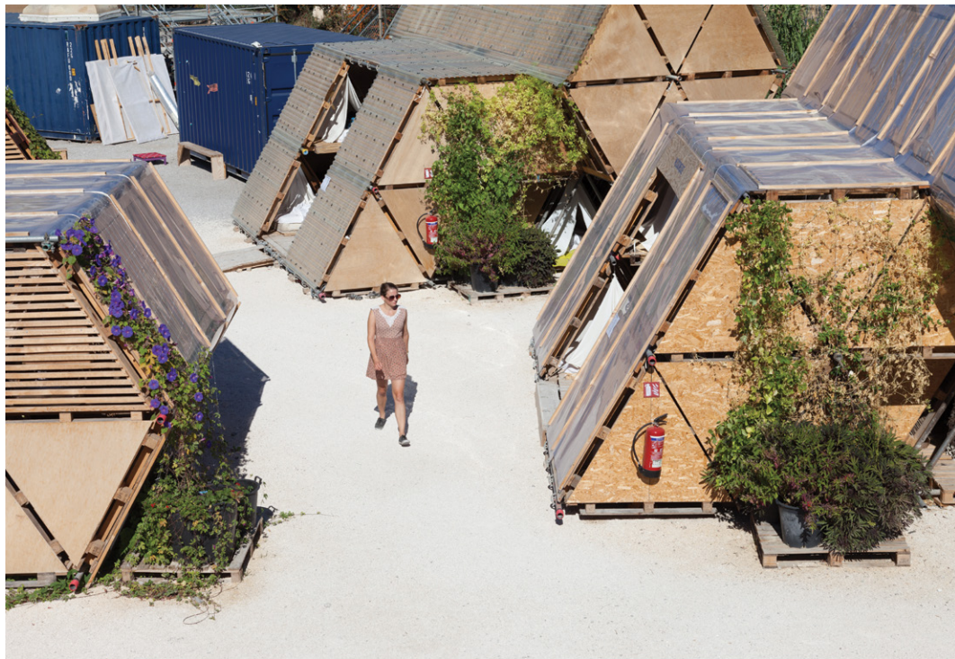
FIGURE 5 'Semeuses' - 'Sowers'. Dorms and small rooms built on scaffolds made out of wooden materials and recycled pallets. Designed by BC Architect & Studios and Michael Lefeber (Photograph by Yes We Camp! 2013).
